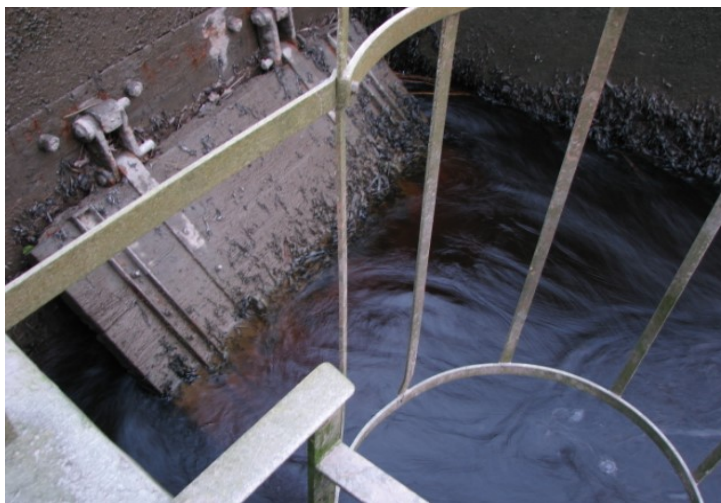
Figure 17: Tidal gate at Arthog, allowing drainage water to discharge into the Mawddach estuary at low tide.
