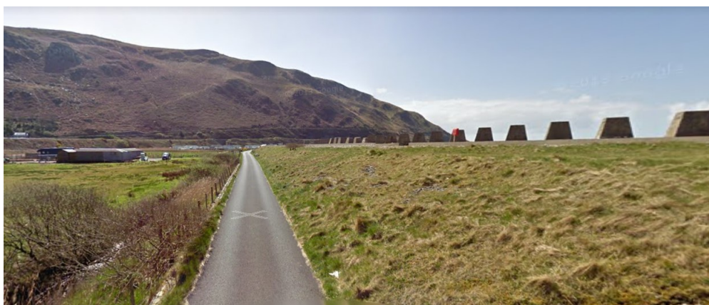
(c) landward slope of the storm beach
