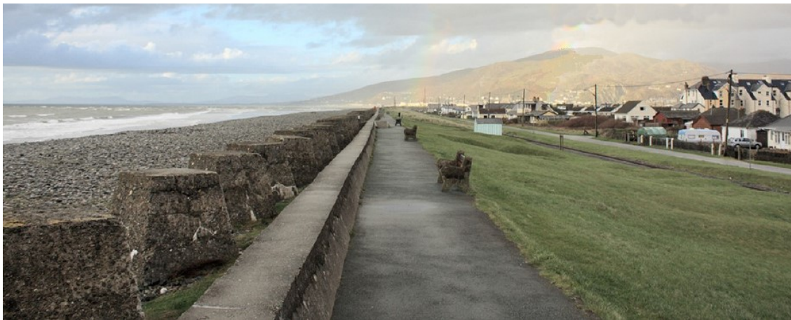
Figure 36: View along the Ro Wen spit, Fairbourne showing the considerable width of the storm beach and landward embankment.
