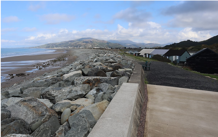
Figure 27 Recently reconstructed sea wall embankment at Friog.
