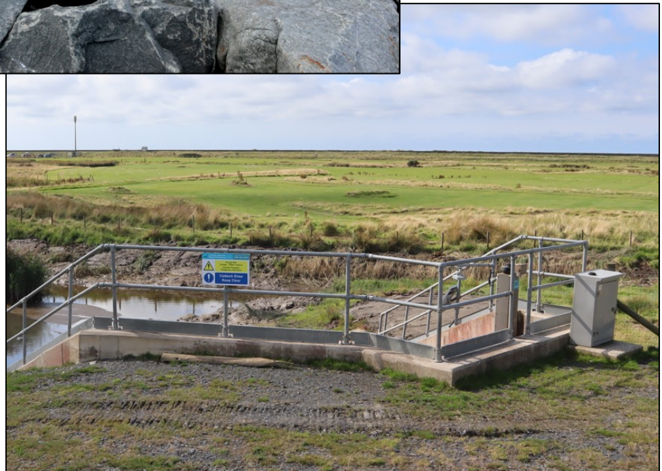
Recent improvements to Fairbourne flood protection. (above) Rock armour added to the storm beach at Friog. (below) New tidal gate at the mouth of the Afon Henddol.
